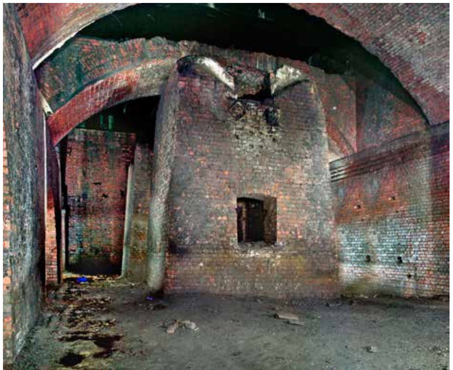
Two wagon hoists at the eastern end, beneath the Central Station goods yard, built around the time of WW1, but not used much beyond that period. Goods could be taken this way to Manchester Docks. Later arching now surrounds the hoists.
